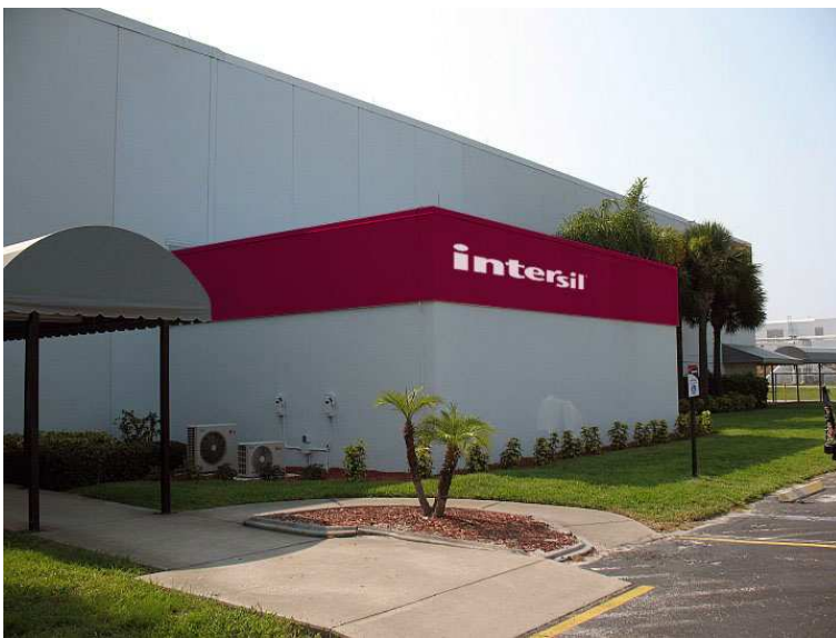
Fig. 6: External view of the completed low dose rate irradiator.
