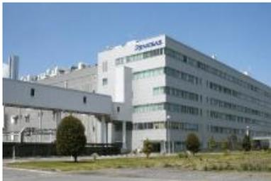
The Naka Site takes charge of the chip manufacturing part in the semiconductor LSI manufacturing flow. The main type of chips manufactured is system LSI. In an effort to meet the increased LSI demand, the Naka Site has enhanced its production efficiency by operating the manufacturing line for 300 mm diameter wafers in addition to the manufacturing line for 200 mm diameter wafers.
