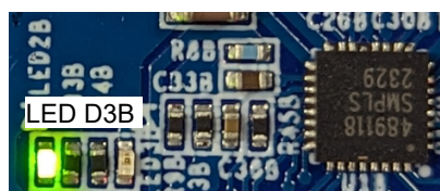
Figure 5. Power Indicator for Source Mode
