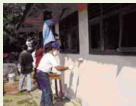
Employees paint a school wall
